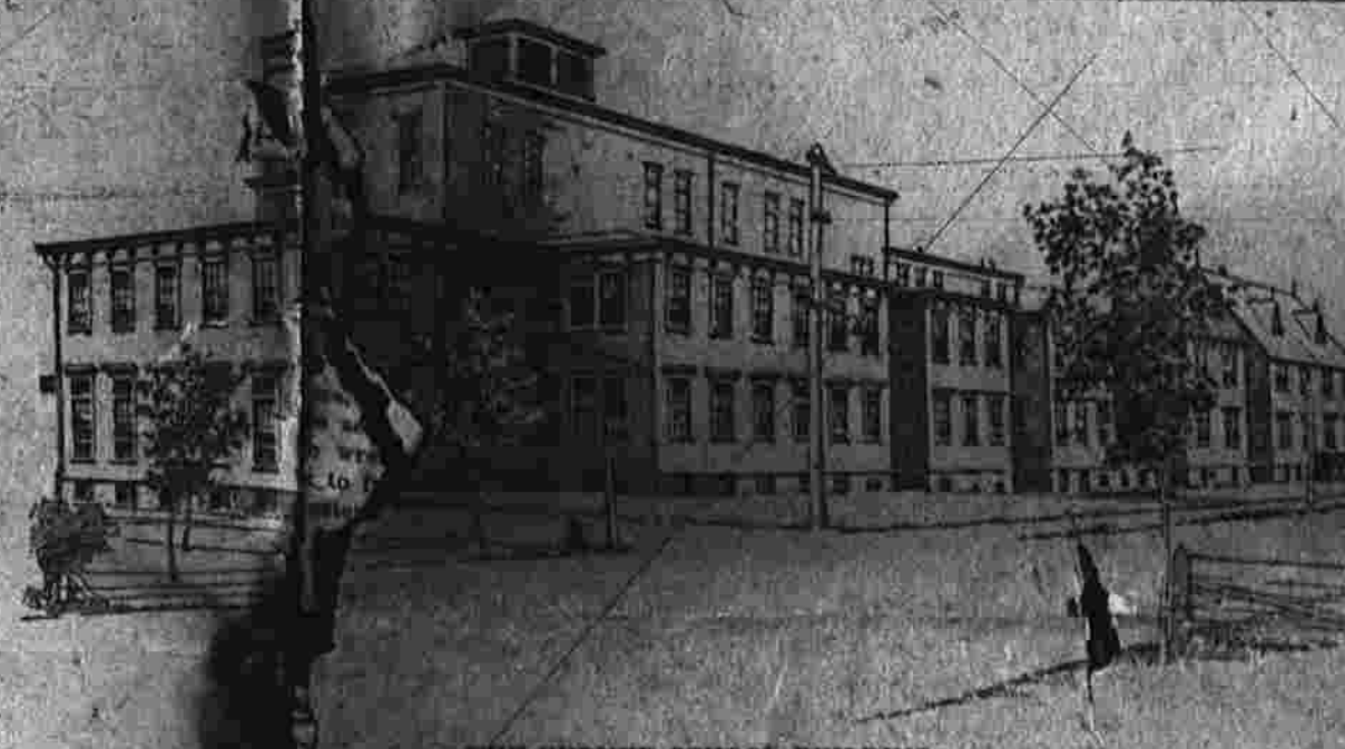
THE BURNED SCHOOL BUILDING.
